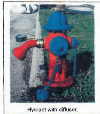
Hydrants with elbows to redirect stream.
